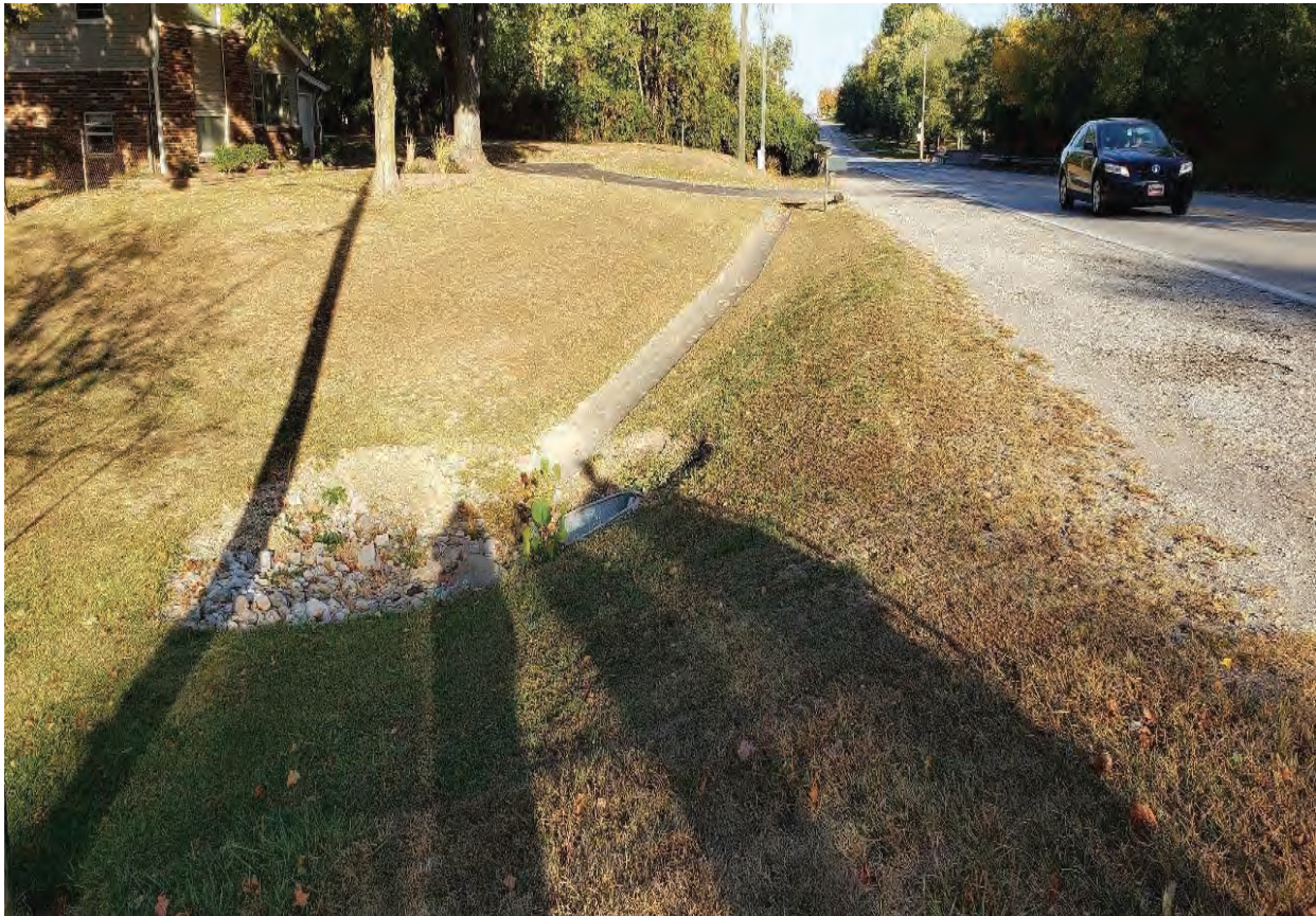
71. Looking east at concrete ditch to culvert
