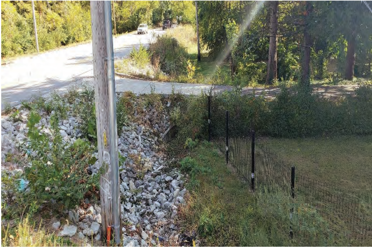
41. Looking east at rip rap roadside ditch to drive culvert draining to UNT 1 to Pleasant Run Creek
