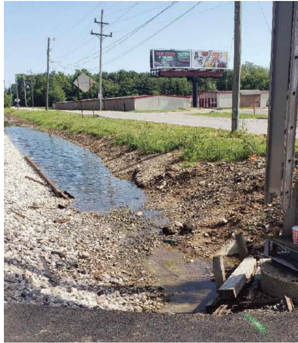
65. Looking north along east side of railroad. Note drainage ditch partially obstructed.
