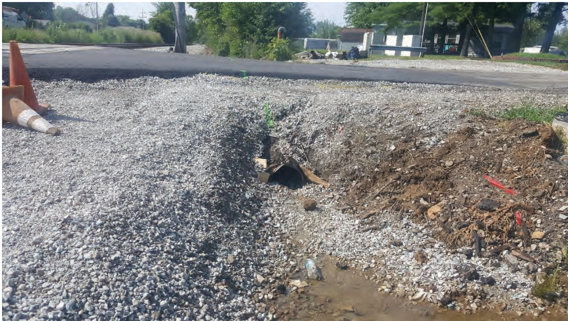
42. Looking south to culvert draining roadside ditch west of railroad and north of County Line Road
