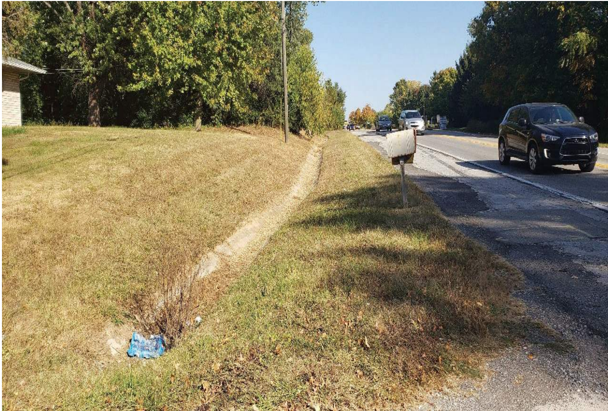
93. Looking east along concrete lined roadside ditch
