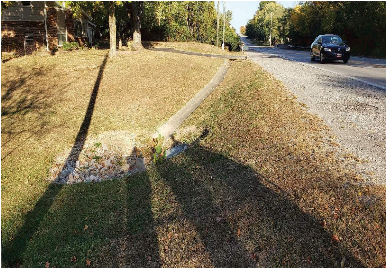
71. Looking east at concrete ditch to culvert
